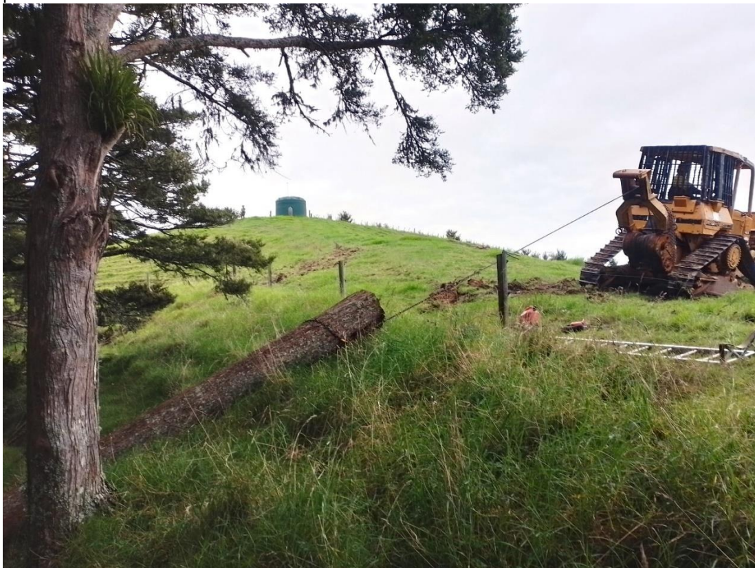
Figure 7 - Michael Harrison expertly winched logs with a TSK D4H Cat without the machine ever entering the forest area.
